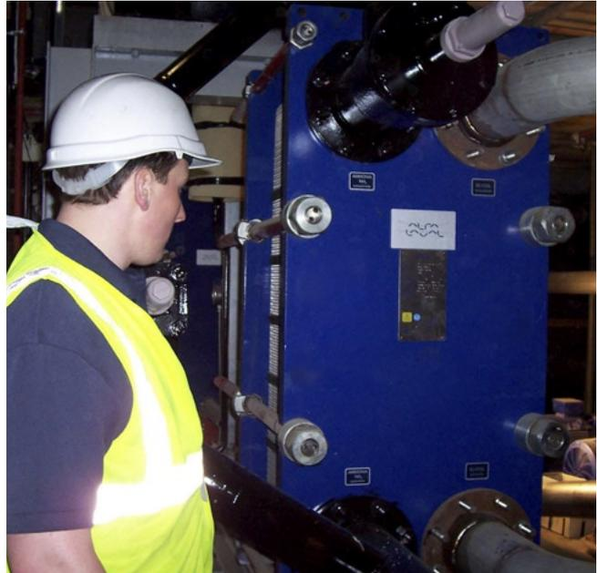
Two plate heat exchangers from Alfa Laval maintain the internal temperature in the produce depot at a constant +2°C.
