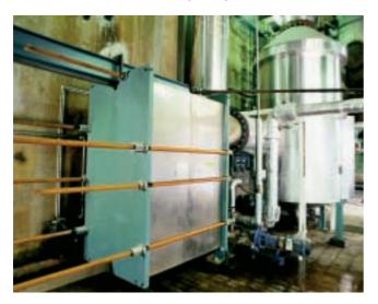
The plate evaporator installed as a replacement for a shell-and-tube evaporator at Kemira AB in Helsingborg, Sweden.
